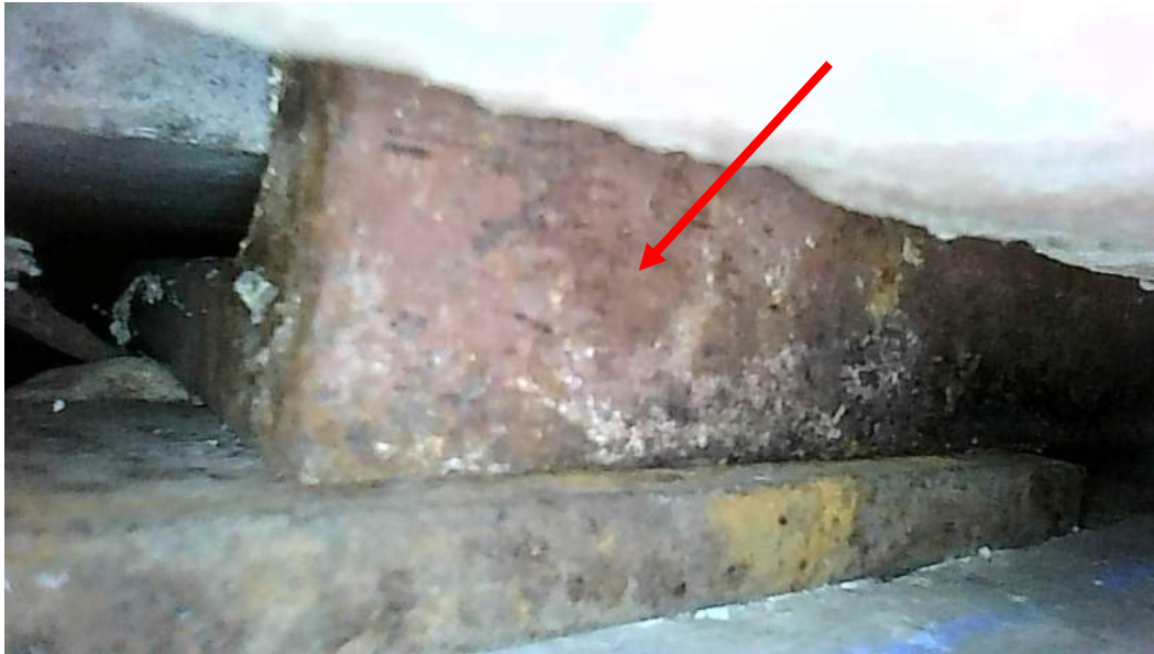
Photograph 3 – Typical support angle at horizontal joints in granite panels.
