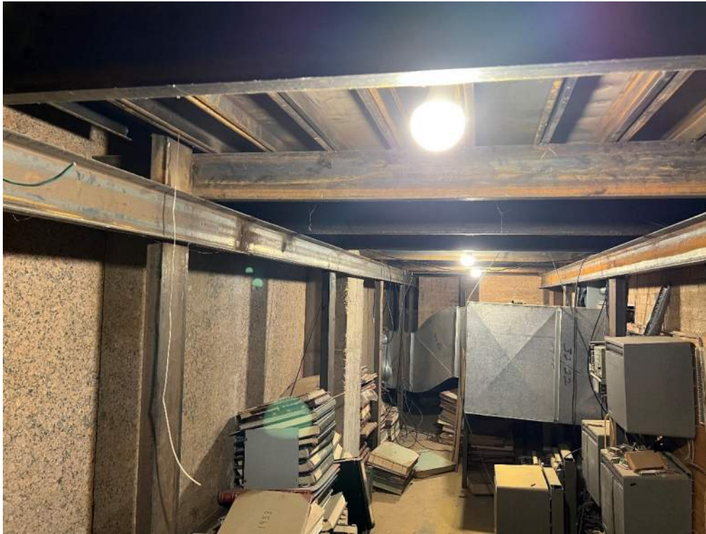
Photograph 1 – Typical construction within storage areas within expanded floors.
