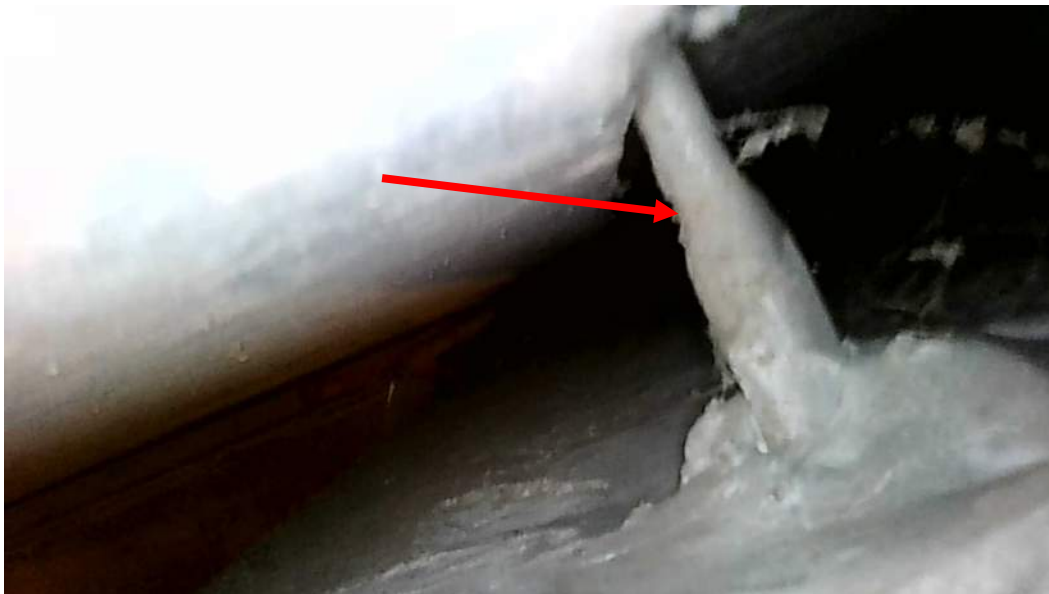
Photograph 4 – Typical lateral restraint anchor at horizontal joints in granite panels.
